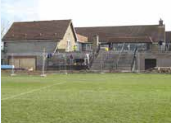
Construction work, April 2012
