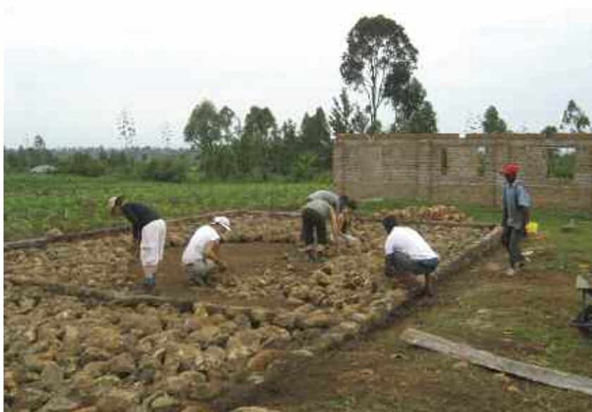
Laying the foundations
