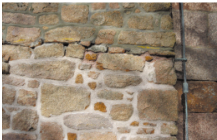
The new lime mortar contrasts with the older, dark cement above it
